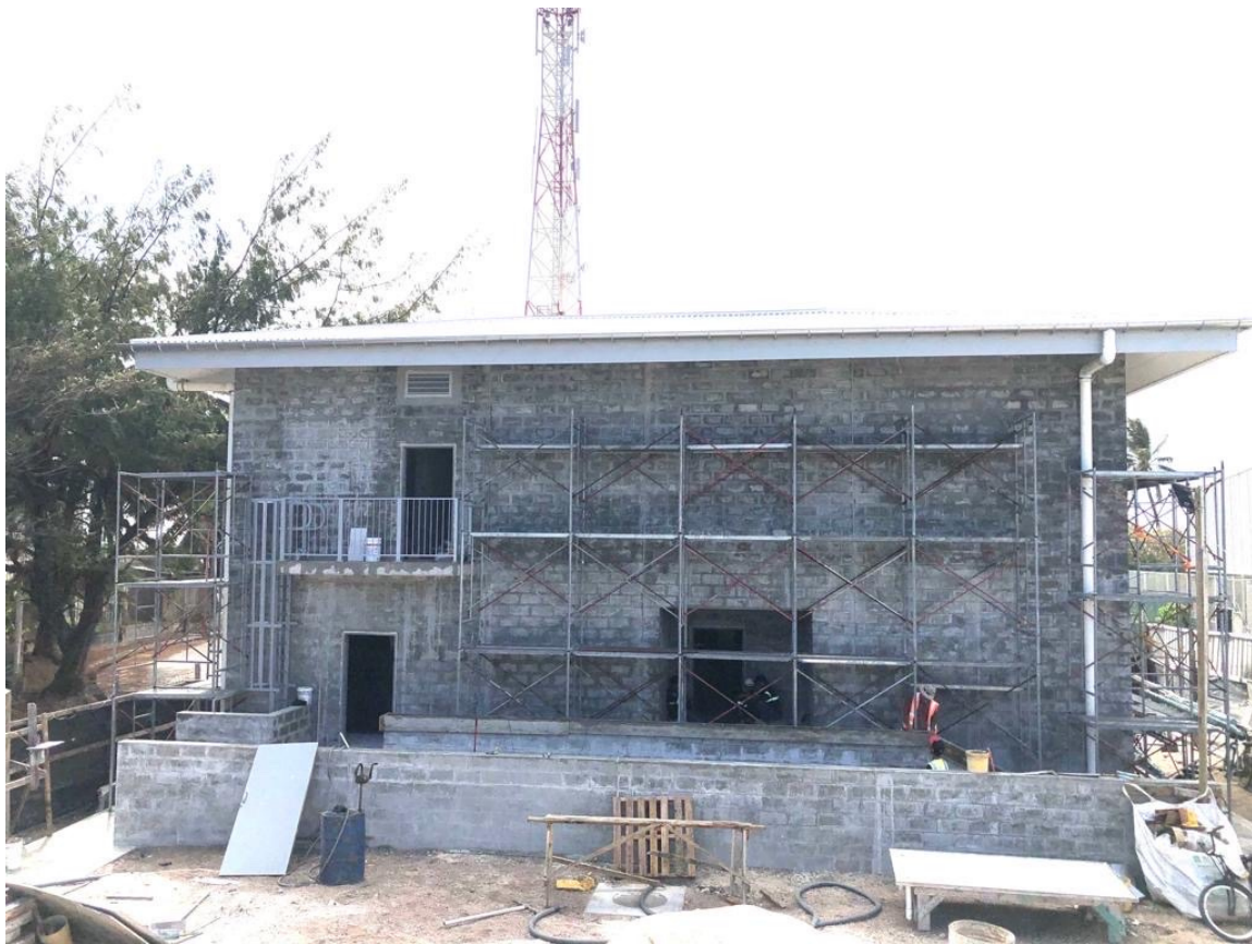
Emergency Operation Center in Ebeye under construction
